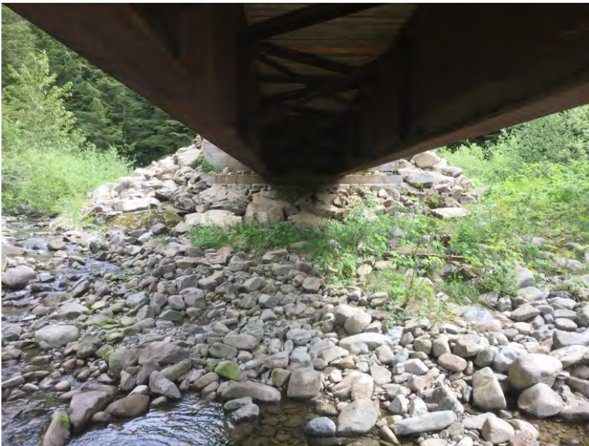
Left Bank Abutment when facing downstream
