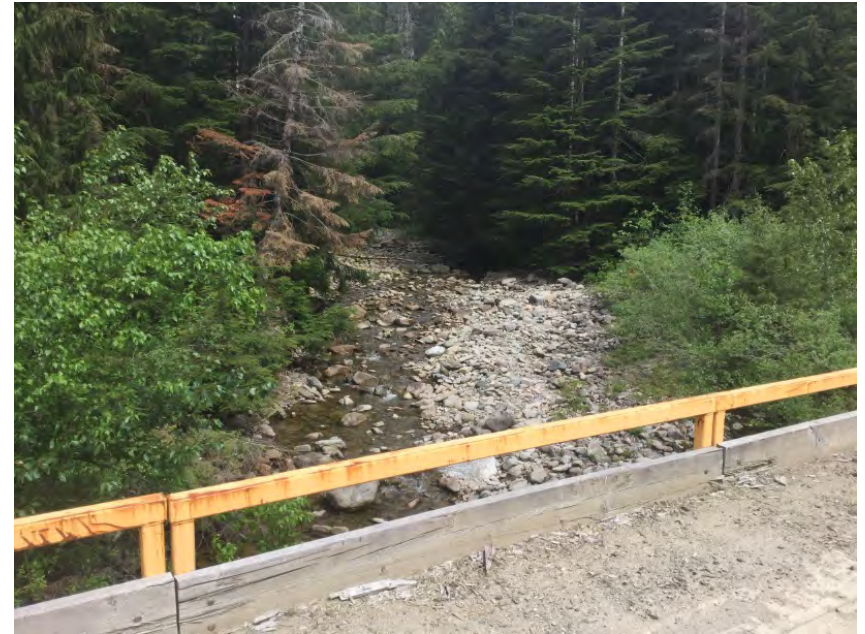
Upstream from Crossing
