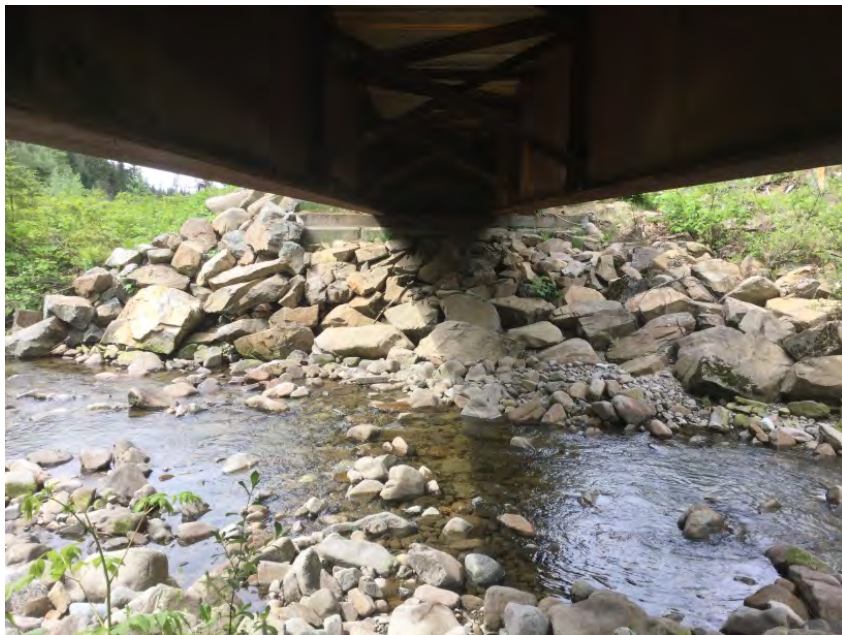
Right Bank Abutment when facing downstream
