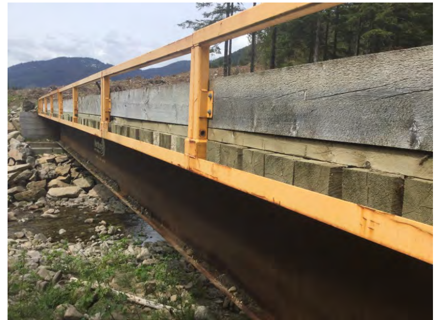
Treated ties and subdeck
