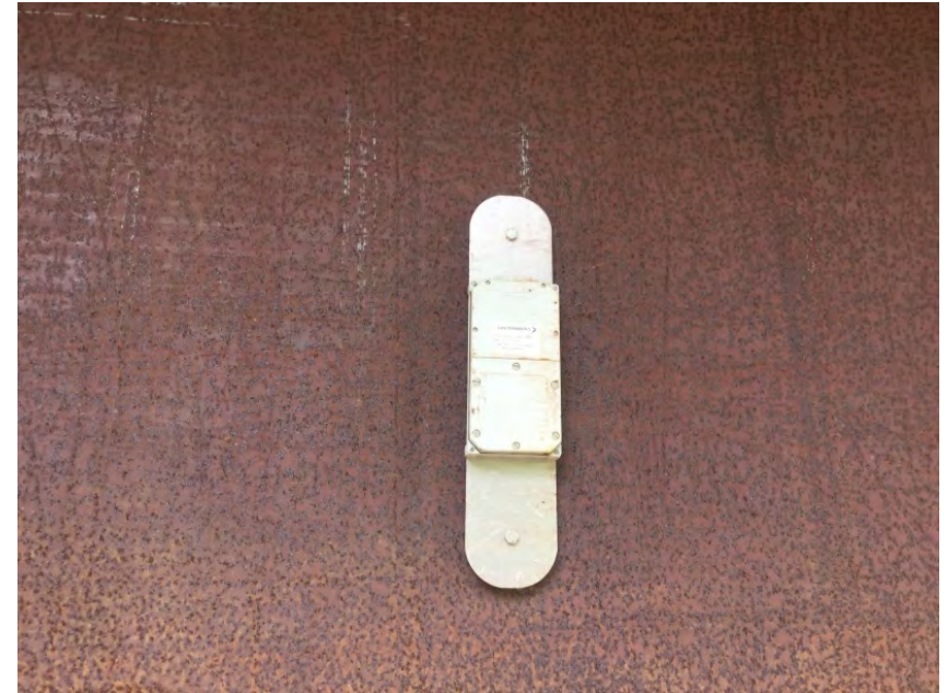
Attached to upstream girder web
